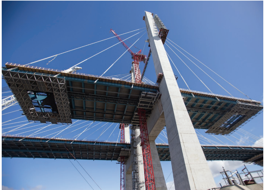
Slag Cement - Tappan Zee Bridge
